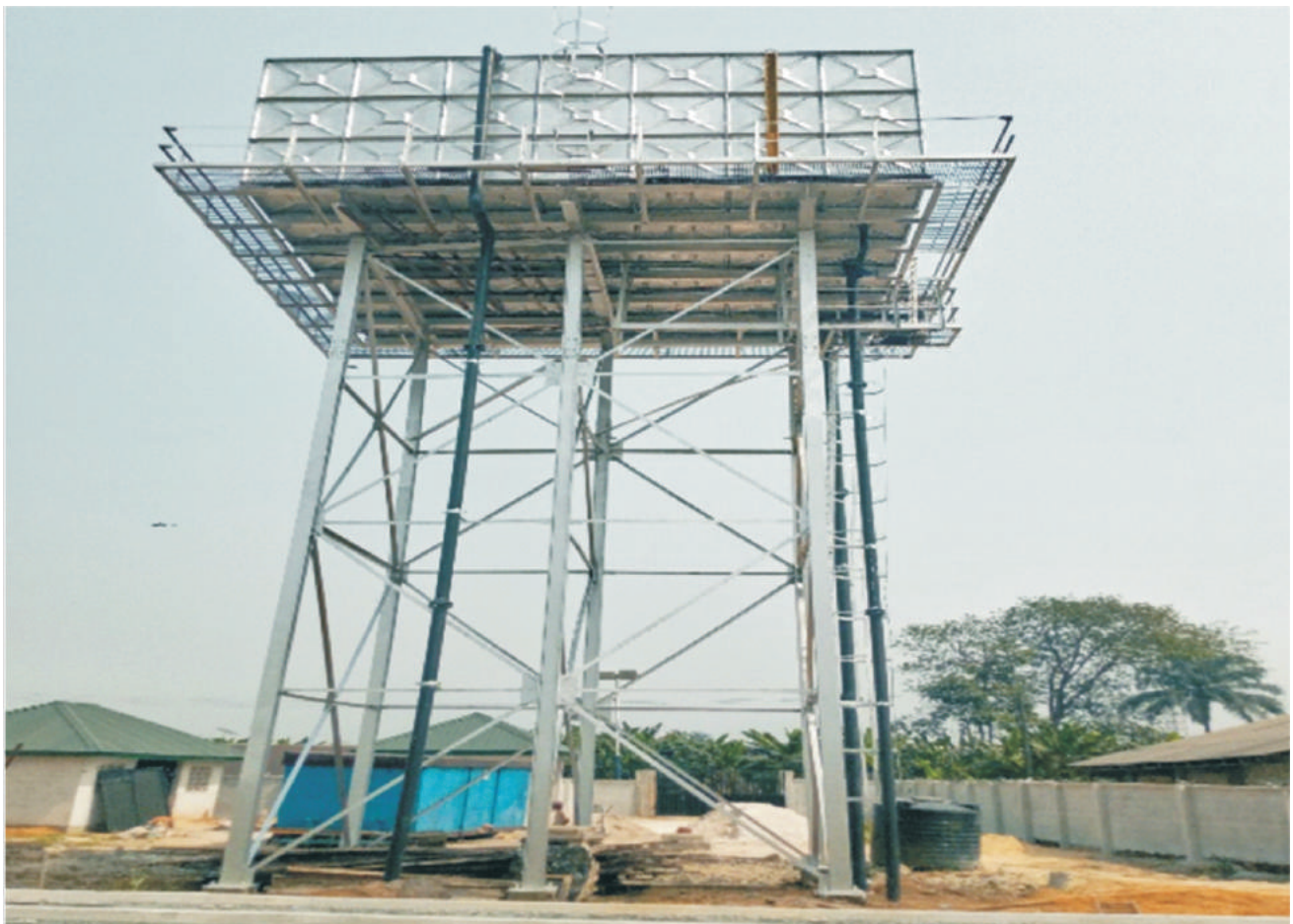
Completed Overhead Tank at Ebulu
