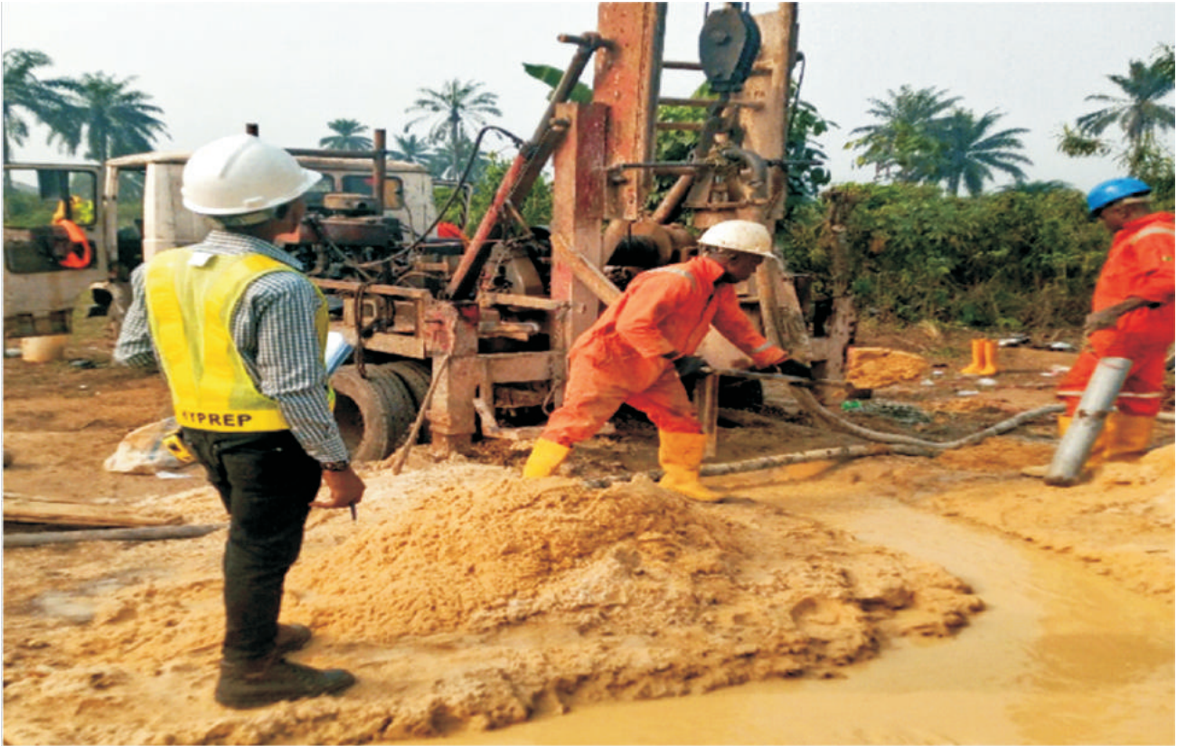
Drilling of Borehole at Ogale
