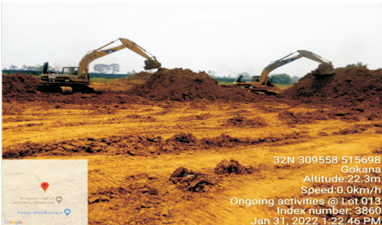
Plate 1.1: Mechanical serial transferring of treated soil from staging area towards the excavated trenches for backfilling in progress at Lot 013, Nweekol Zorbuke, K.Dere, Gokana L.G.A.
