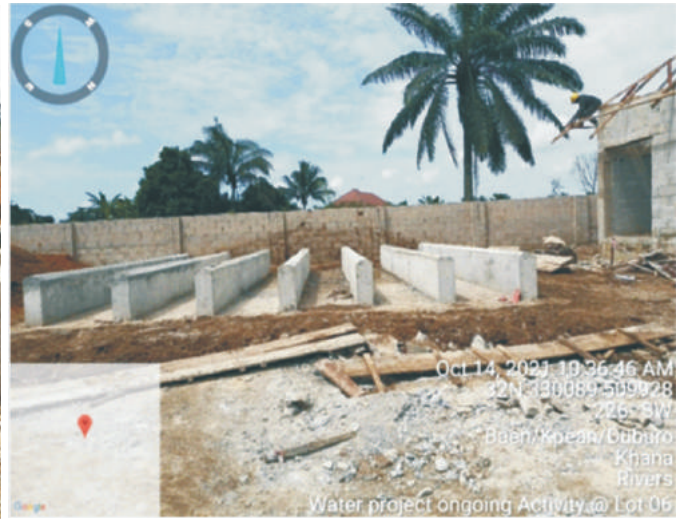
Treatment House and Ground tank foundation under construction at Kpean
