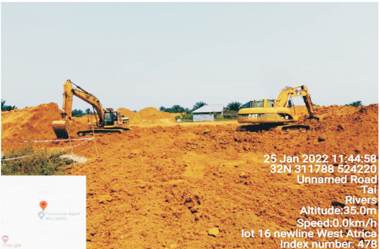
Plate 1.3: Mechanical transferring of excavated impacted soil towards the engineered biocell for treatment on-going at Lot 016, Buemene Korokoro Well 05, Tai L.G.A. (Contractor: NEWLINE WEST AFRICA LTD)
