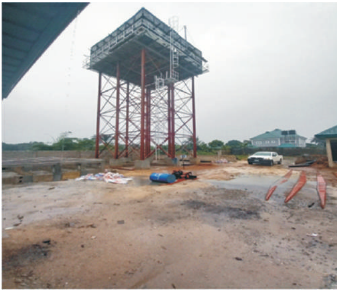
Constructed Overhead Tank at Korokoro
