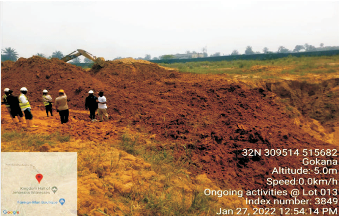
Plate 1.2: HYPREP Operations Unit Remediation Supervisors on routine inspection of on-going backfilling process in progress with Contractor's Site Personnel and Community Workforce Representatives at Lot 013, Nweekol Zorbuke, K.Dere, Gokana L.G.A. (Contractor: CENTENNIAL DEVELOPMENT & INVESTMENT LTD)
