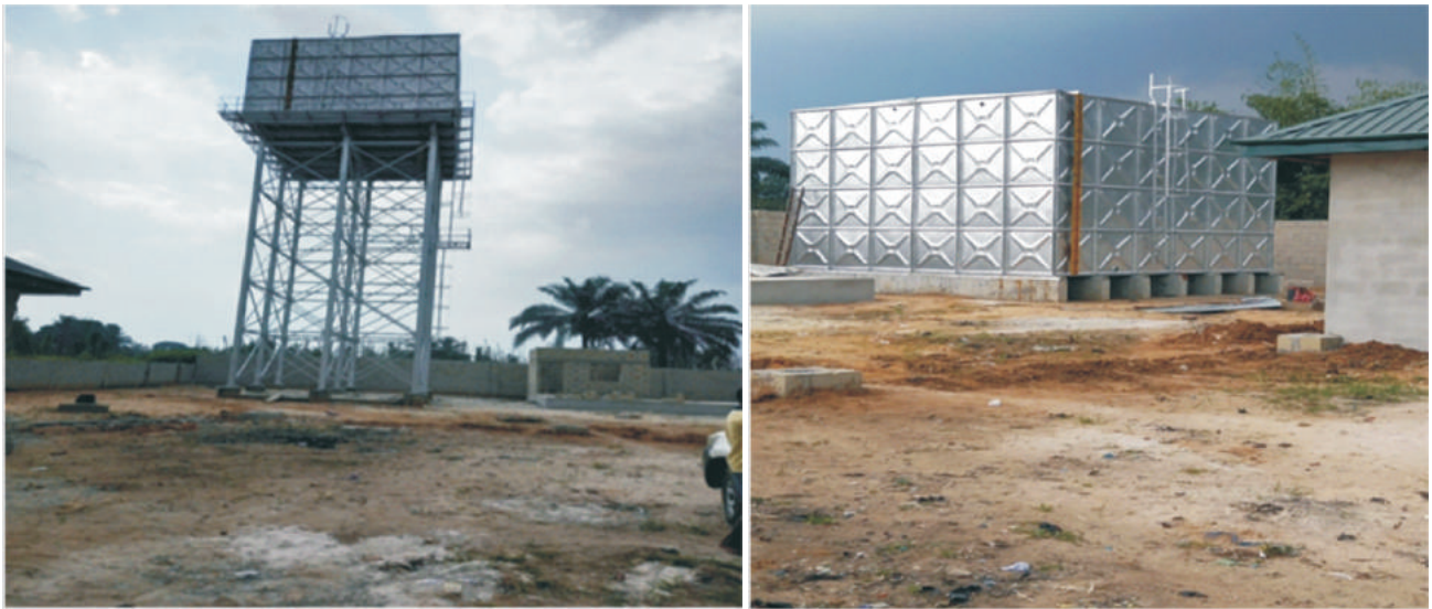
Constructed and installed Overhead and Groundwater Water Tanks at Barako Water Station
