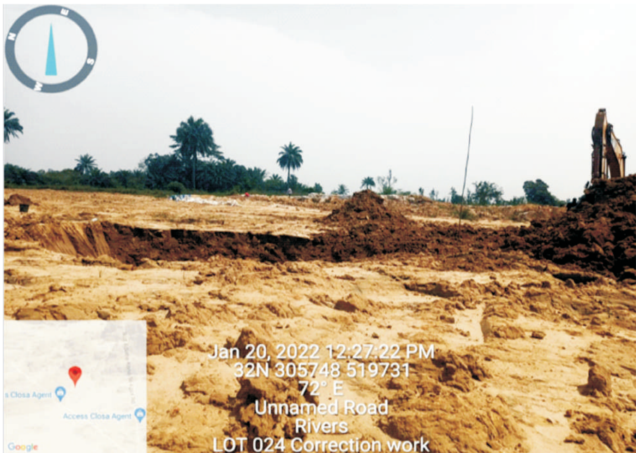
Plate 1.4: Correction of exceedances (retrieval and re-treatment of samples which had higher TPH values than target closure limit from NOSDRA Close-out results) at Lot 024B.Dere / Gio, Gokana / Tai L.G.A. Remediation Contractor-LEVENE ENERGY DEVELOPMENT LTD.
