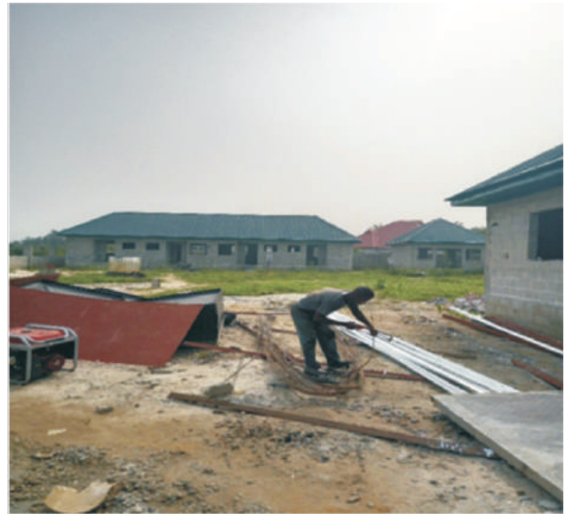
Ongoing Construction of Treatment house at korokoro
