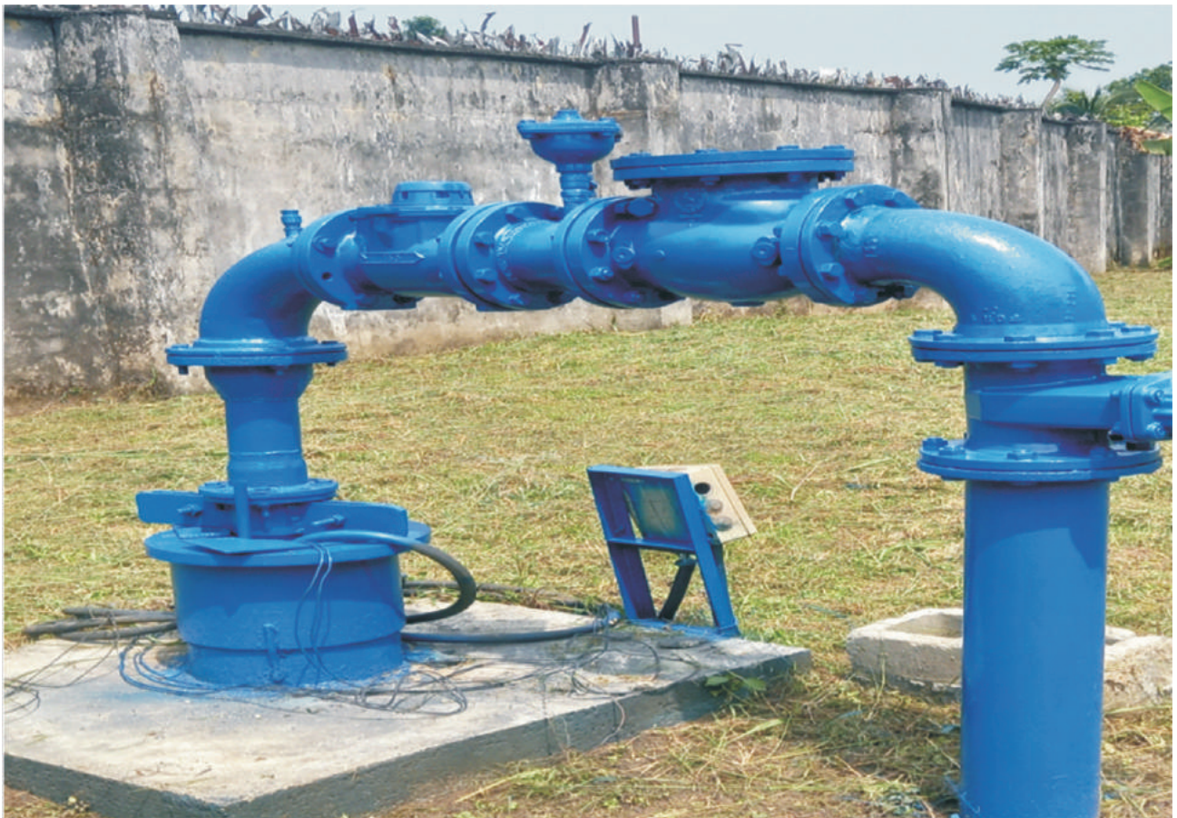
Completed and installed Borehole Head at Terabo
