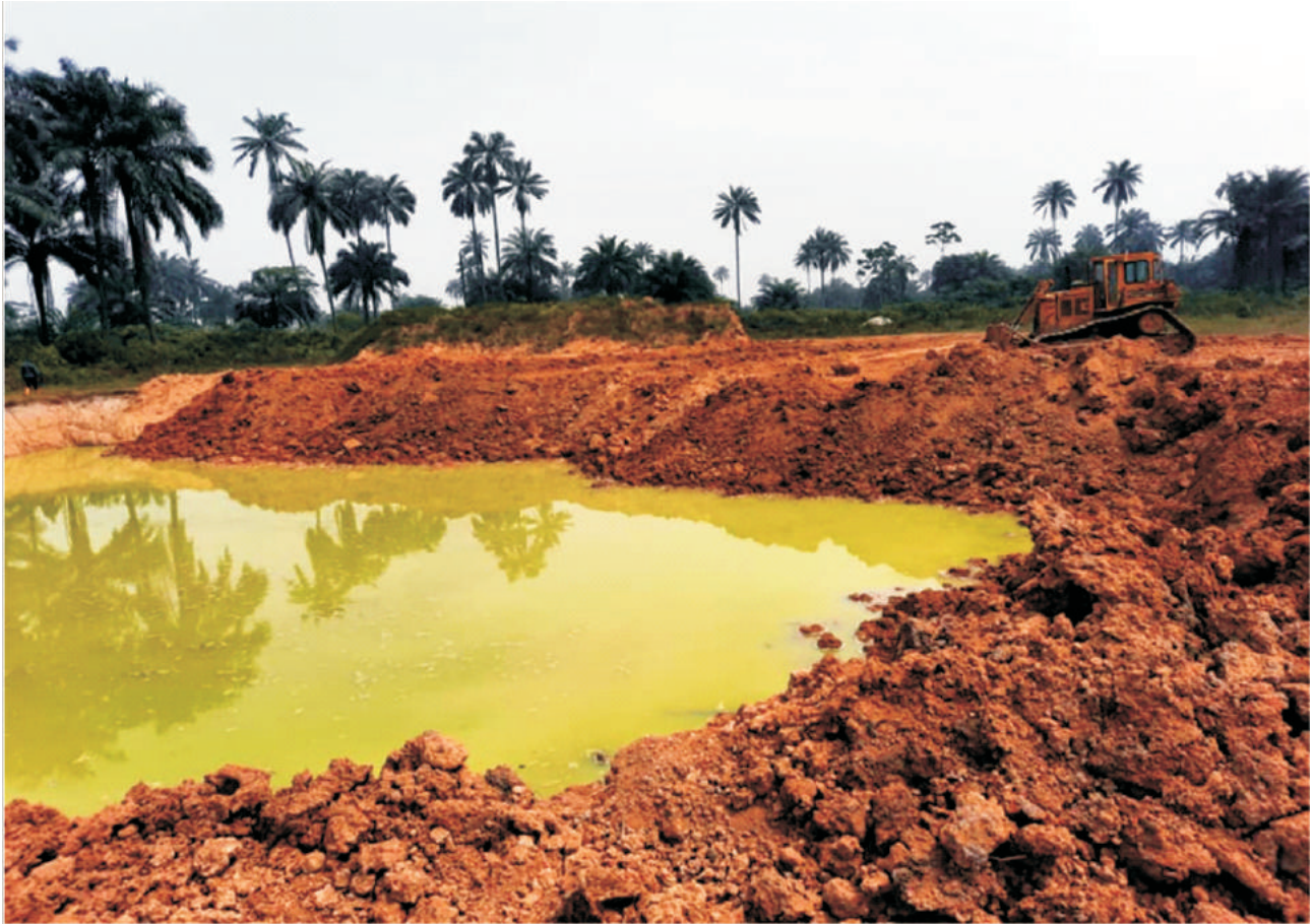
Plate 1.5: Backfilling of excavated pits with treated soil in progress at Lot 046New Elelenwa Manifold, Akpajo, Eleme L.G.A. Remediation Contractor - ANDELSTA LTD.
